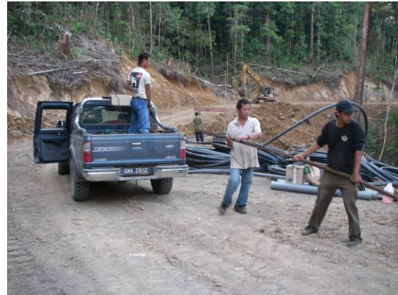
Samling employees delivering water pipes to Long Benalih (19-20 August 2007)
